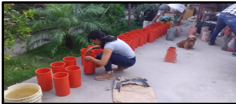
Figura 3.13: Engrasado de moldes
