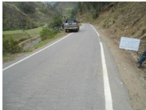
Figura34Tramo Km 85+000 - Km 86+000
