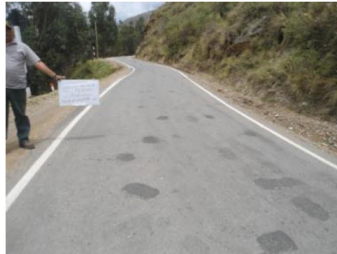
Figura31Tramo Km 82+000 - Km 83+000
