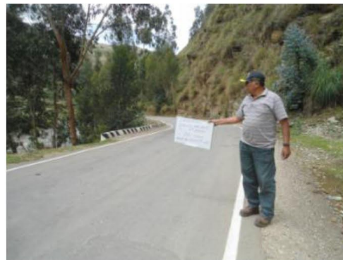
Figura36Tramo Km 87+000 - Km 88+000
