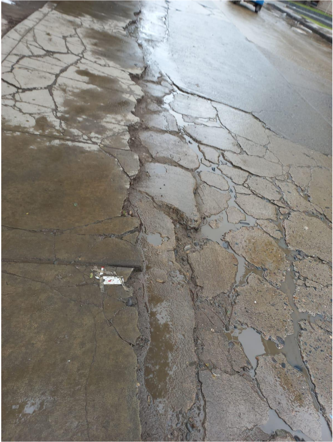
Berma colapsada
